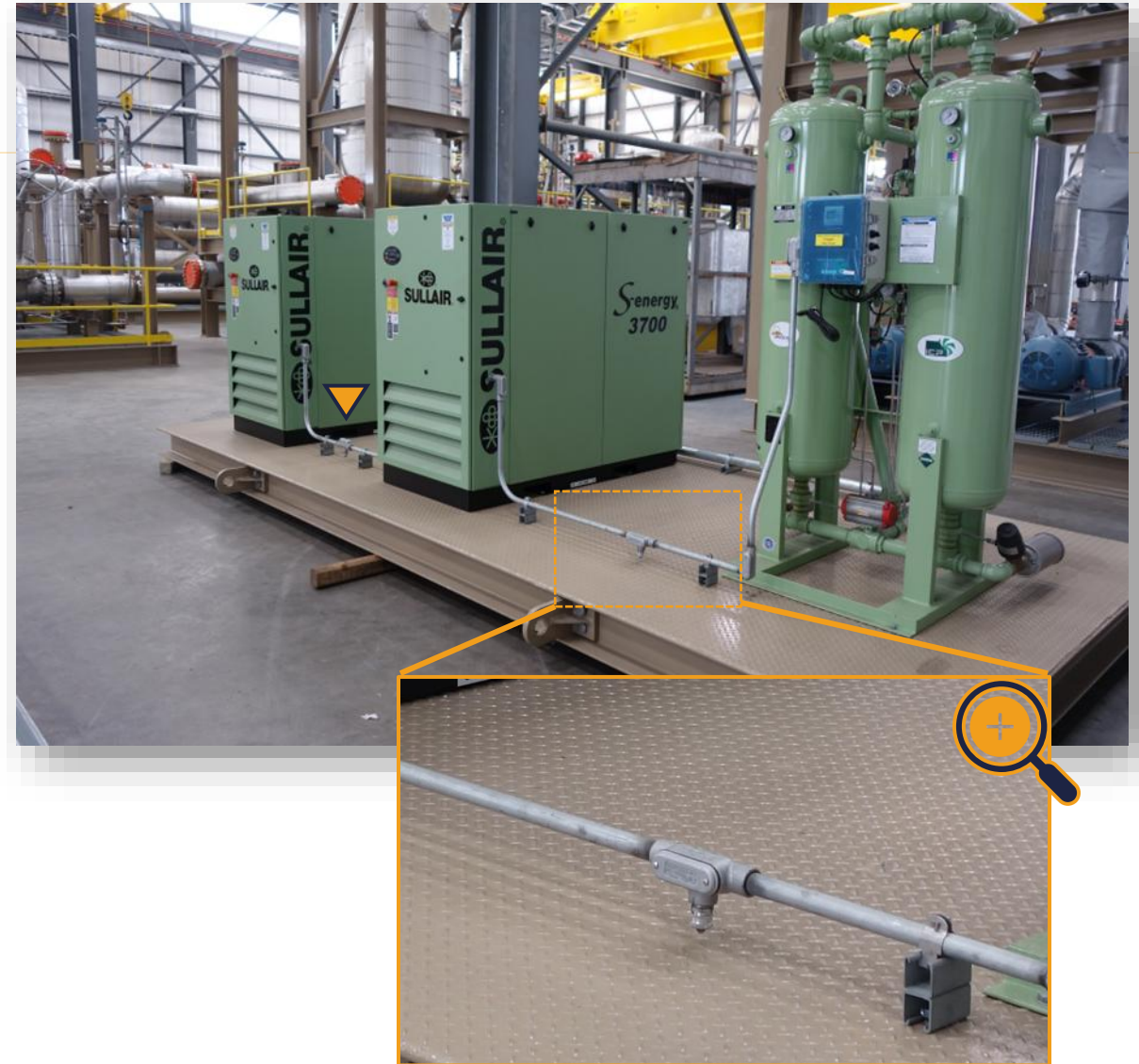
Drain fitting installations
